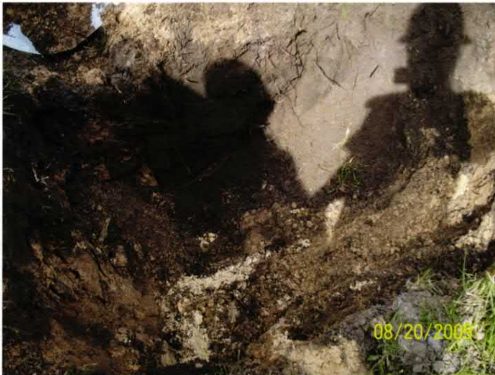
Picture 2: Excavation after tank removal.
